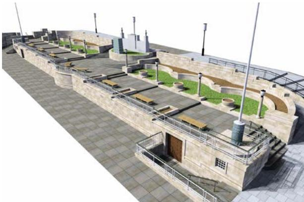
To facilitate replacement of the roof deck, the scheme required careful removal, storage, refurbishment and relaying of the existing pavings, stone works and balustrading. The scheme also required Planning and Listed Buildings consent and the design team worked closely with the local conservation officer as well as English Heritage and other stakeholders to achieve a successful outcome.
